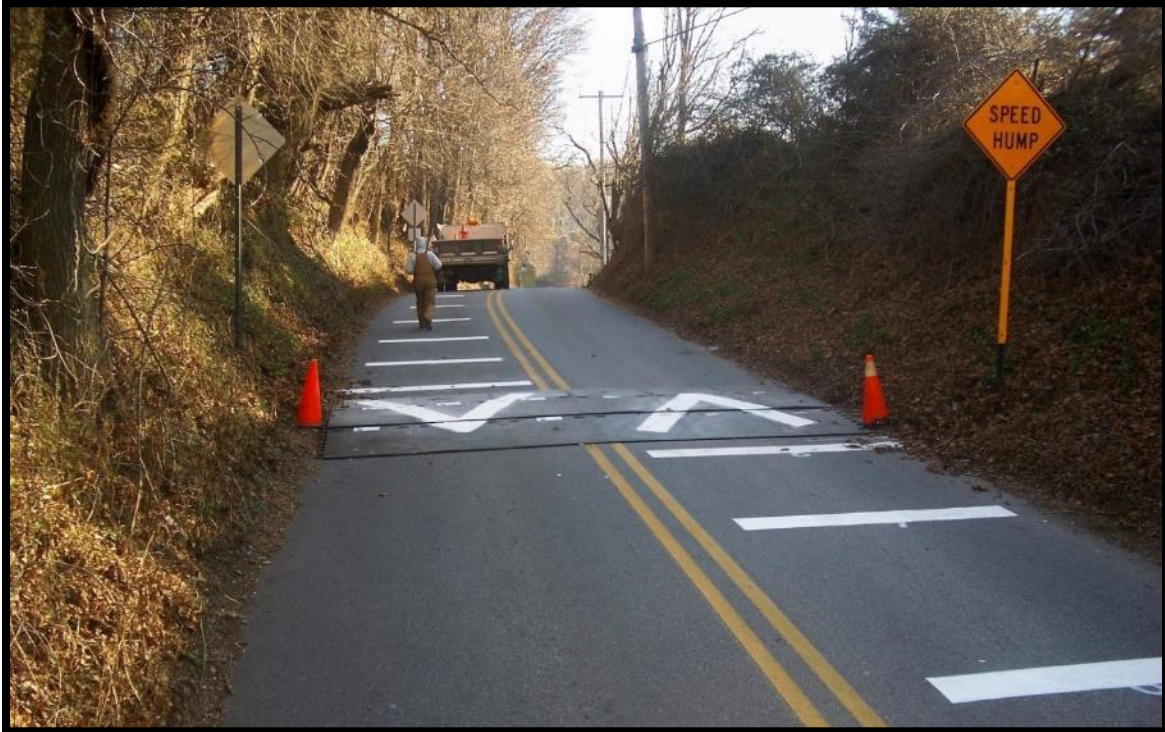
Figure 6: Example of a Temporary Speed Hump
